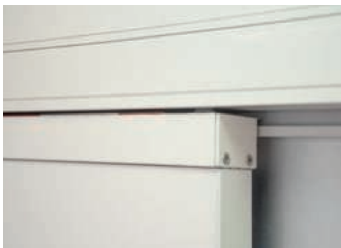
Top door leaf connected to operator
